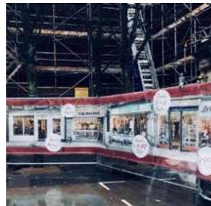
Museum repair work covers supporting businesses affected
